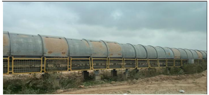
Exhibit 6: 4.5km conveyor belt (OLBC) from mines to plant
