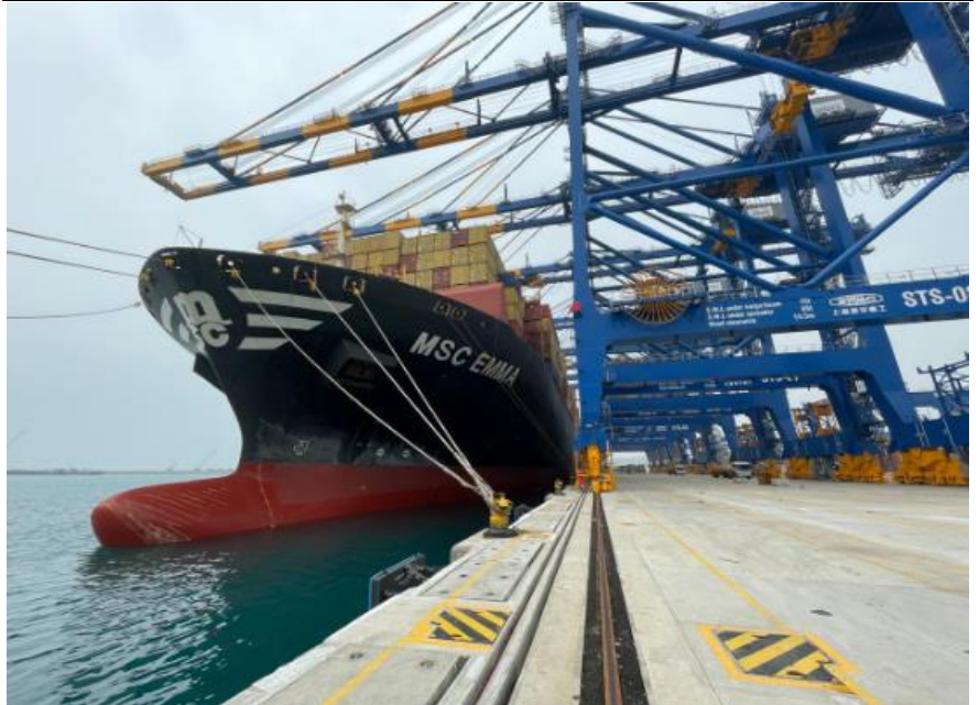
Exhibit 5: 800m berth in Phase 1 capable of handling largest vessels in the world
